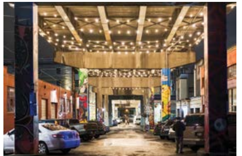
The Central Eastside Viaduct Lighting Project transforms key gateways with long-awaited safety improvements. Photo by Dustin Pattison Photography.
