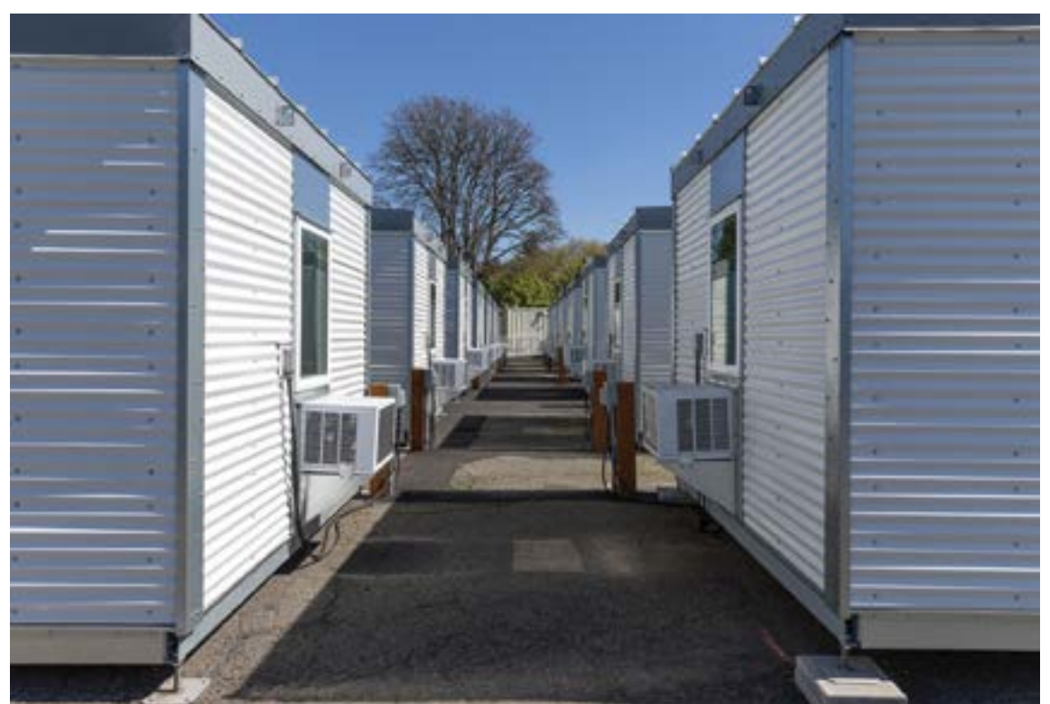
Harrison Community Village units. Photo by Multnomah County.
